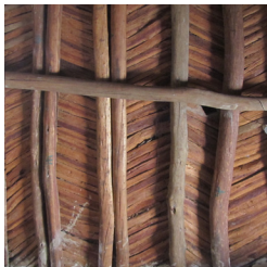
WOODEN ROOF the roof adaptes the local way of construction with the exclusion of the mud.
